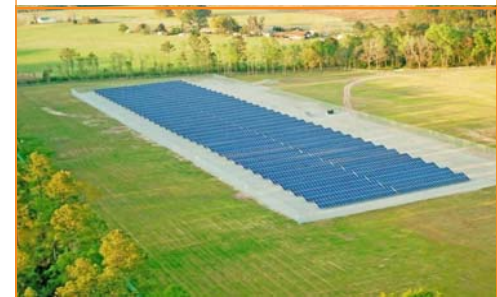
Birdsong Peanut Company – Colquitt, GA 1 Megawatt Solar Array – Ground Mount
