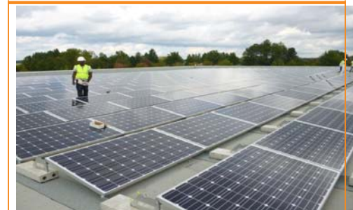
Hewlett Packard Data Center – Suwanee, GA 350 kW Solar Array – Roof Mount
