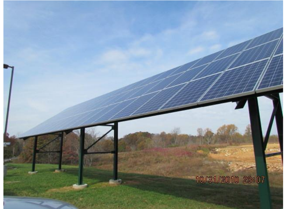
J&S Construction– Putnam County 37.5 kW ground mount
